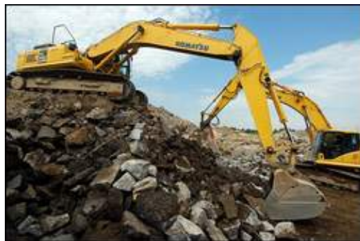
John Huff/Staff photographer Excavating equipment reclaims material from The Rochester Shoppes site off the Spaulding Turnpike in Rochester, which will be crushed into various types of gravel and reused.
